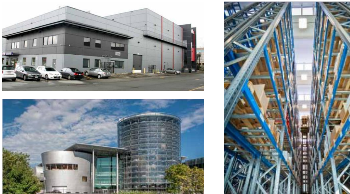
Top: Multi-level industrial building in Surrey, UK, with light industrial use on ground floor and flex space and parking on upper floor – an example of a building with higher floor area ratio yet conventional site coverage. Bottom: Modern transparent vehicle factory in Germany. Right: Modern warehousing and logistics facility with high ceilings. Source: ‘Summary report: Opportunities for the Intensive Use of Industrial Land’, Metro Vancouver, 2013, < www.metrovancouver.org/planning/development/EconomyIndustrialLands/EconomyIndustrialDocs/OpportunitiesForIndustrialLandsIntensification-Feb2013RevisedFinalTitle.pdf >
